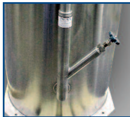
Vacuum-jacketed valve for efficient liquid withdrawal. (half-inch inner pipe)
